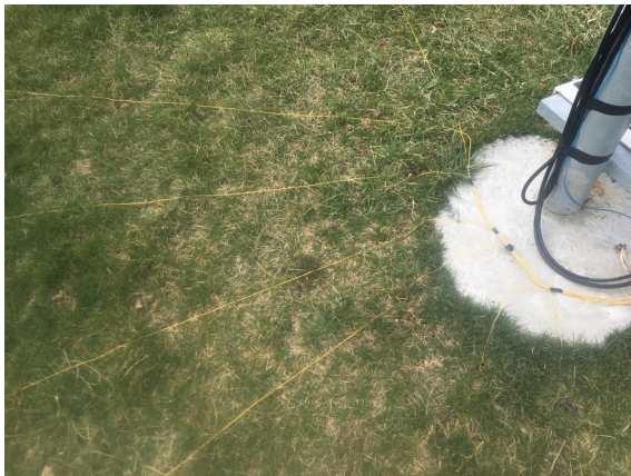
Radials At Base of Tower
